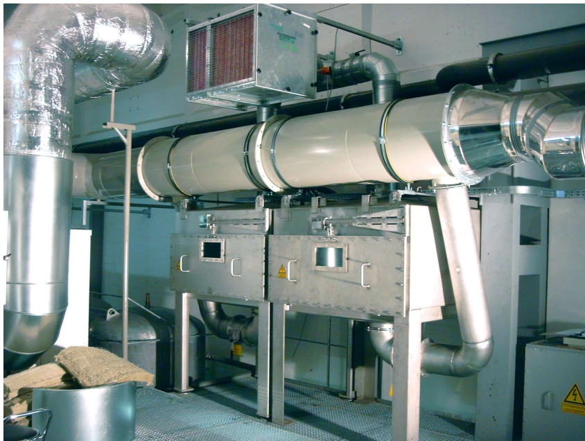
Non-thermal plasma unit of a plasma-catalytic air cleaning system
